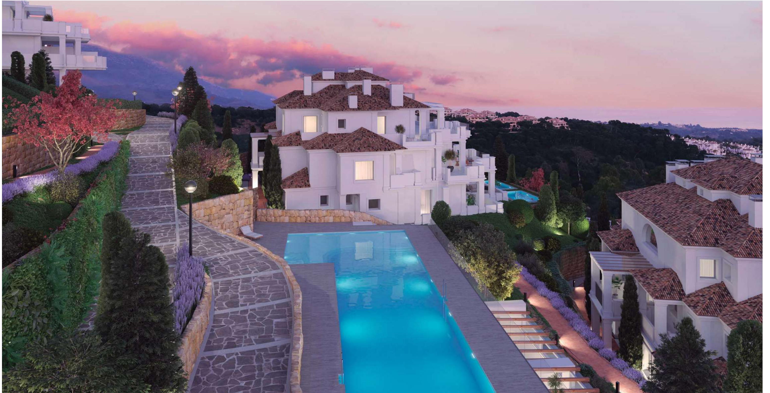
WATCH THE SUNSET FROM ONE OF THE TWO COMMUNAL OUTDOOR SWIMMING POOLS
